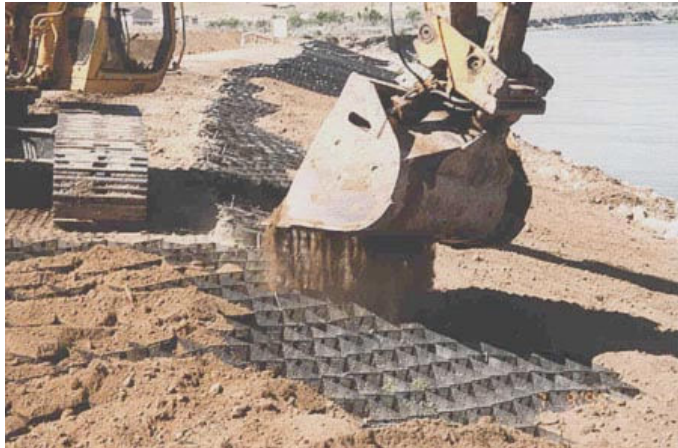
Geogrids being filled with sand for bank protection (IECA photo)
